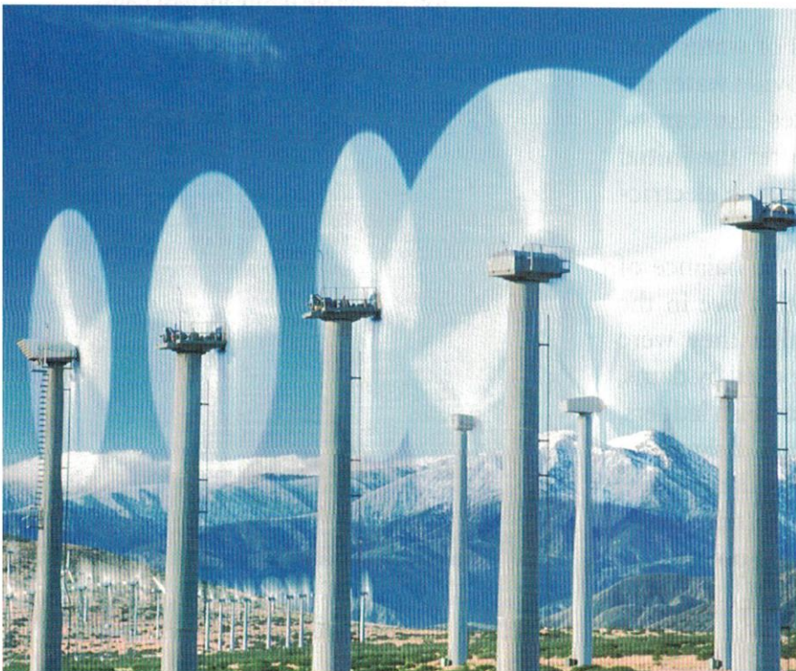
Figure 24 Wind energy is converted to electricity as the spinning propeller turns a generator.
